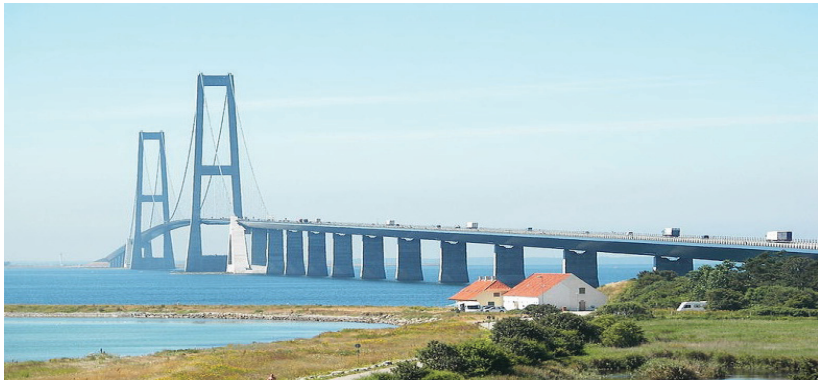
1.22 pav. Great Belt tiltas Danijoje ( http://en.wikipedia.org/wiki/File:Denmark_Great_Belt_Bridge_East.jpg )
