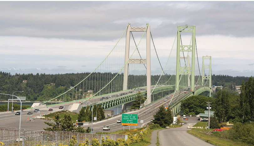
1.20 pav. Westbound Tacoma Narrows ir Eastbound Tacoma Narrows tiltai JAV ( http://en.wikipedia.org/wiki/File:Tacoma_Narrows_Bridge_2009.jpg )
