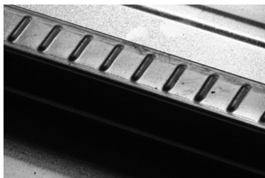
Fig 1. The embossments of the profiled steel sheeting
